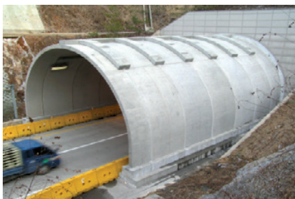
Tunnel extension - Hyeongok (South Korea)
