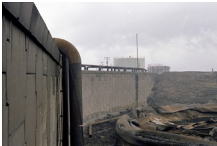
After the oil tank fire - Tacoa (Venezuela)
