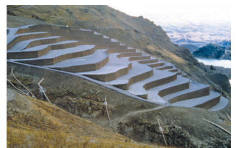
Stabilization of landslide - Cairnmuir (New Zealand)
