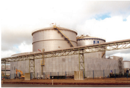
Containment dikes for ammonia tanks - Montoir (France)
