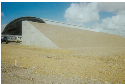
Blast barrier - Townsville (Australia)
